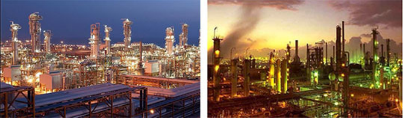
Images of refineries in Assaluyeh
